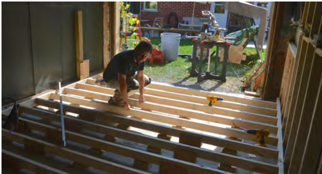
Alexandre Guertin-Pasquier prepares the floor structure of the laboratory's new space.
