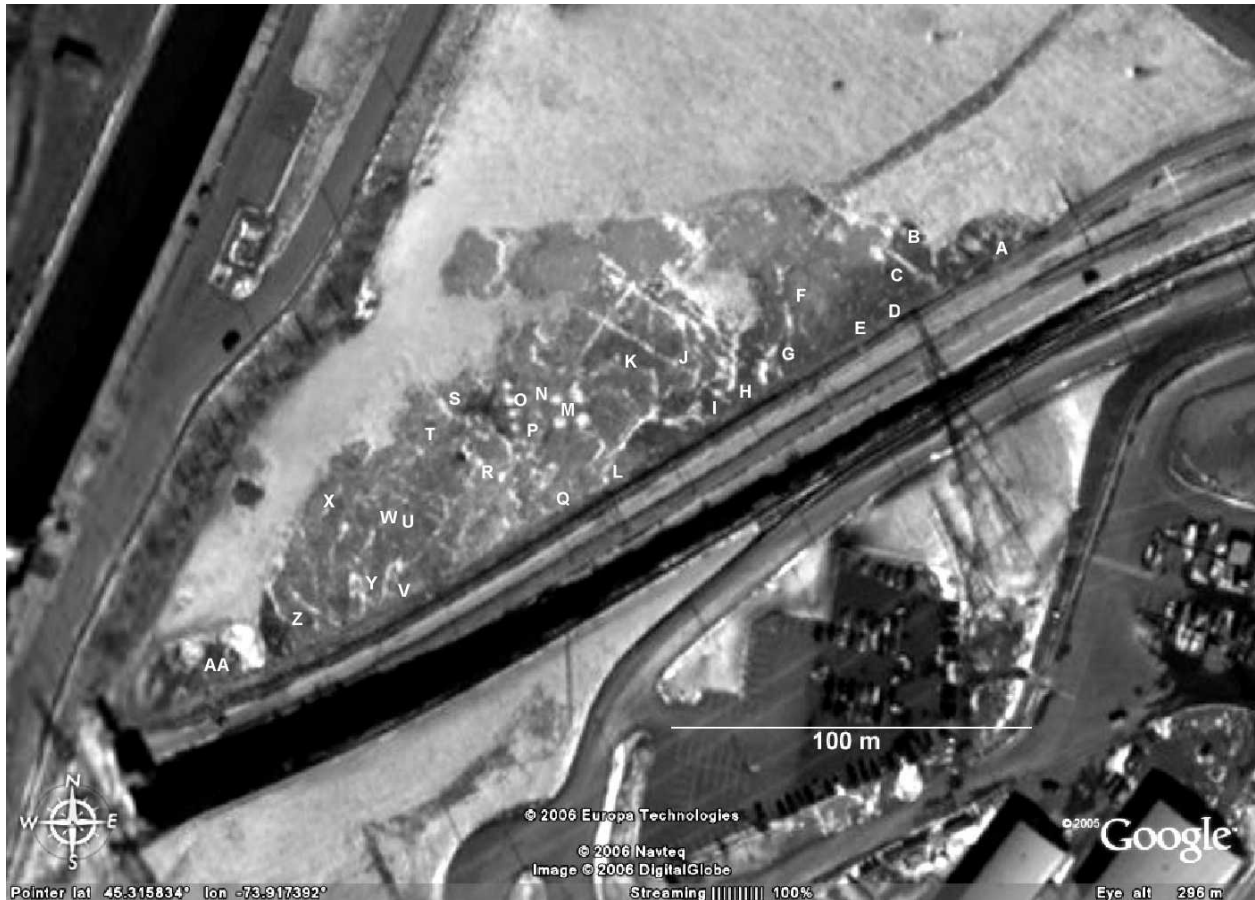
Figure 24. Outcrop along Hwy 132 at eastern entrance of tunnel under St. Lawrence Seaway locks (base from Google Earth)
